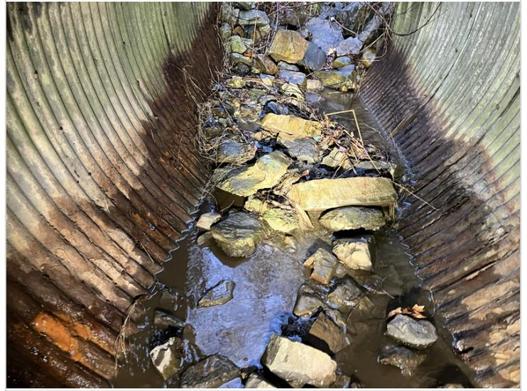
Rock buildup near Upstream End of Culvert
