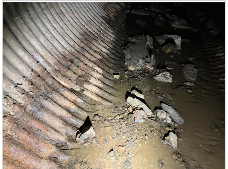
Slight Separation between sections of culvert near
